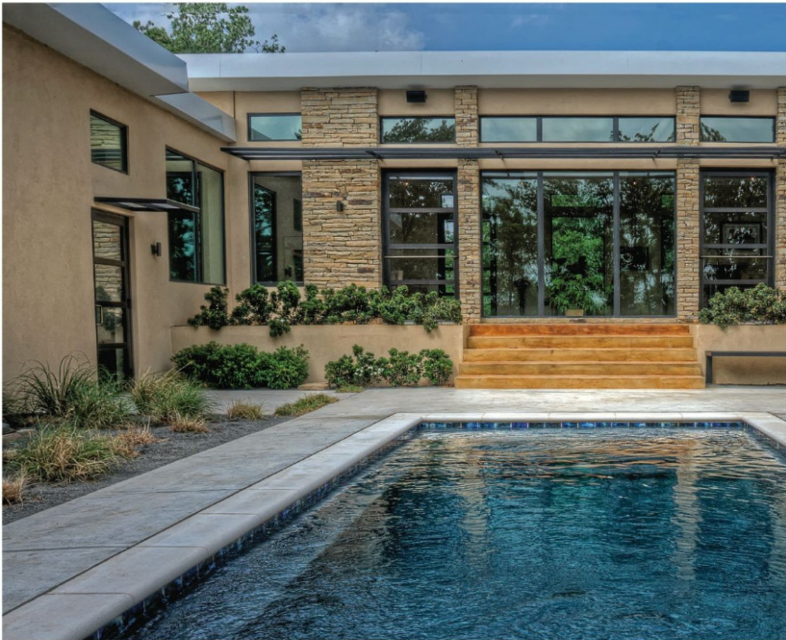
The two rectangles housing the master suite, office, garage and guest areas are perpendicular to the main rectangle, creating a large "U" shape that forms a three-sided barrier around an outdoor living space with a rectangular dipping pool and hot tub.
